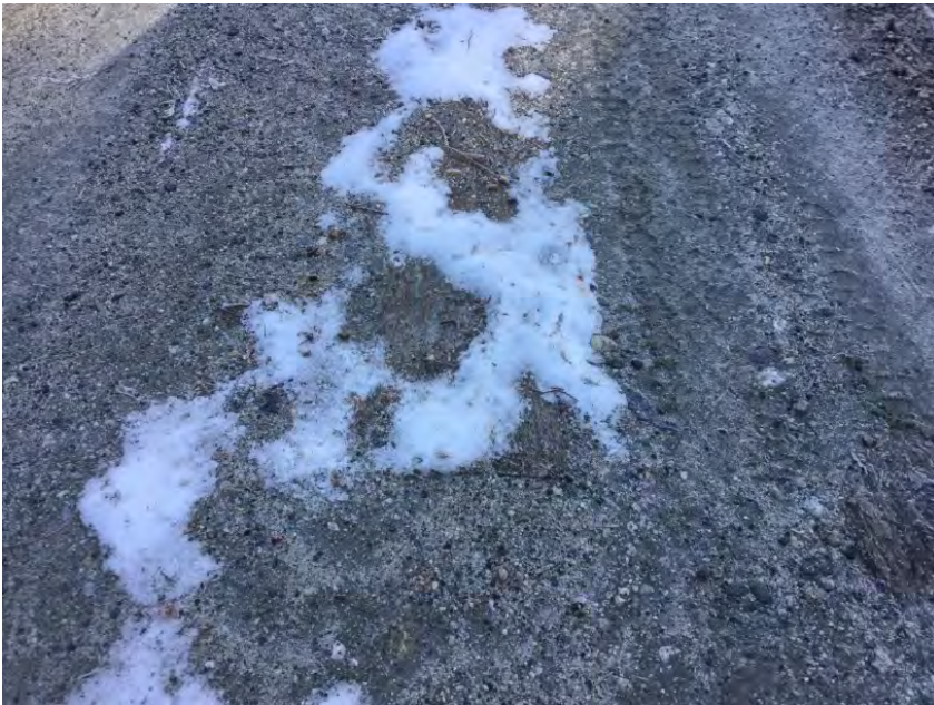
Top layer of stringers visible from surface
