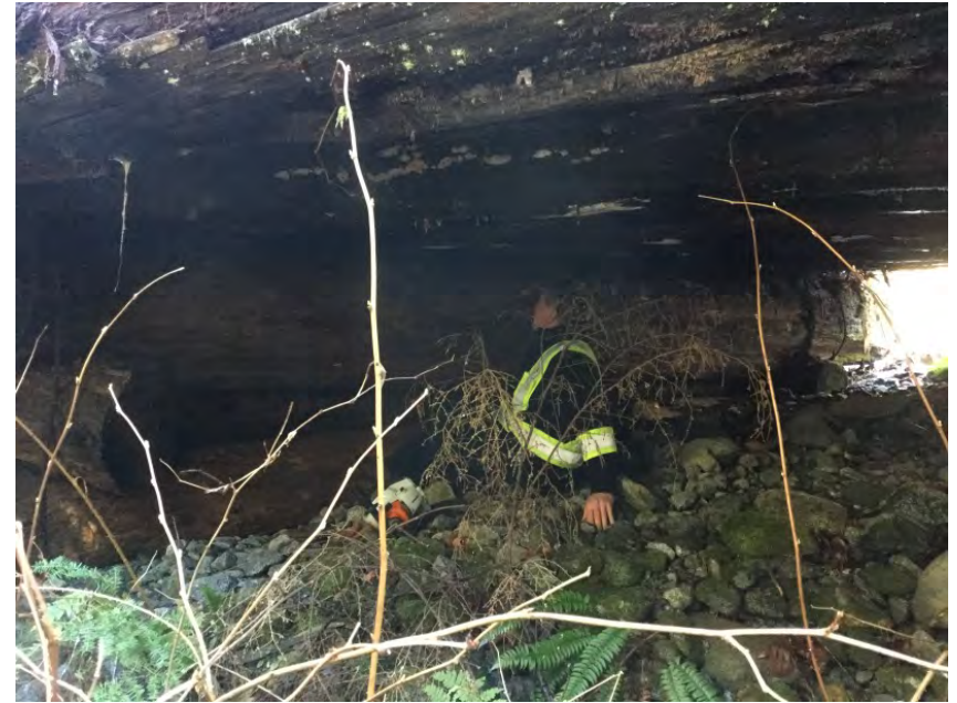
Right Bank Abutment when facing downstream
