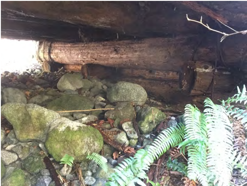
Left Bank Abutment when facing downstream
